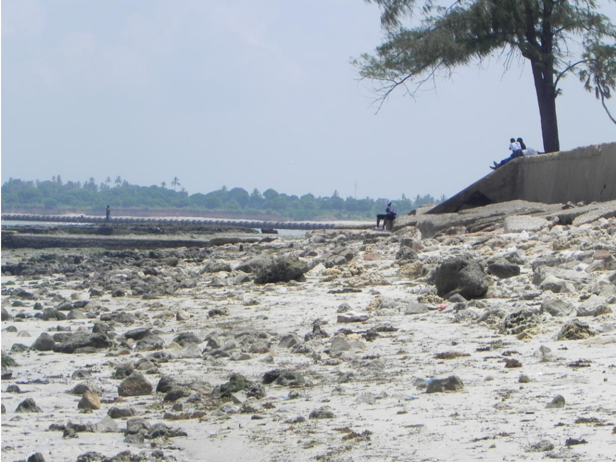
Figure 5: Evidence of water movement towards the wall
