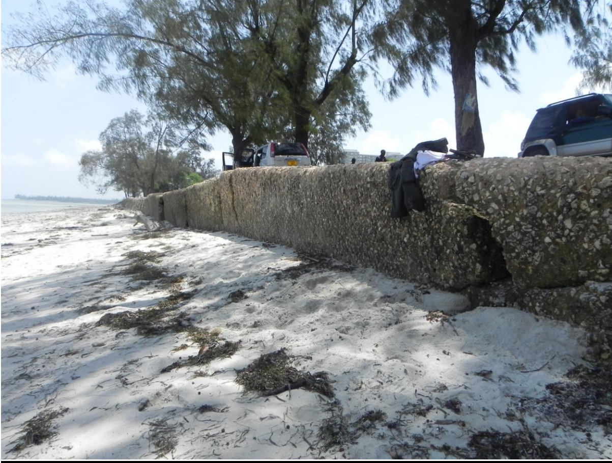
Figure 4: Current Situation Of The Sea Wall In Dar Es Salaam To Be Re-Constructed
